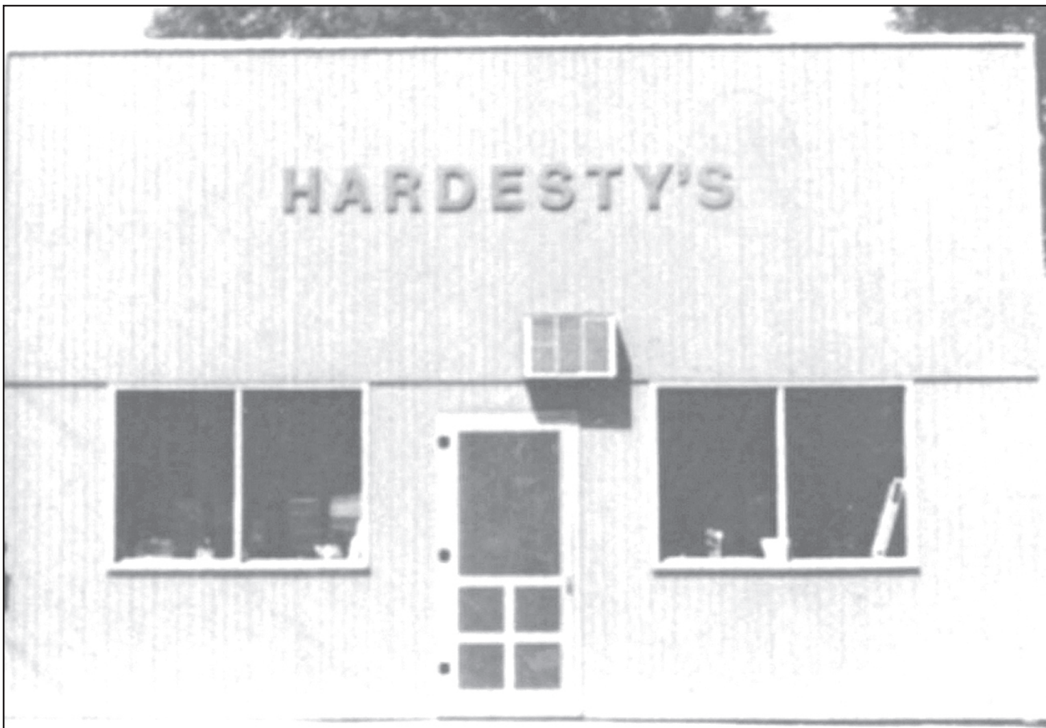
THE OLD HARDESTY DRUG STORE still stands in Jennings as a reminder of the many years it served the town with prescription drug and fountain services. It was also home to the Hardesty family for a time.
