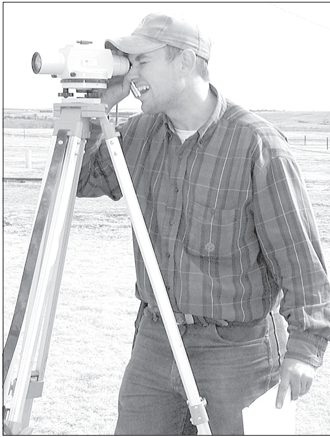
ON SATURDAY Michael Wasson used survey equipment at the Decatur County Fairground to start the leveling work for the new arena and livestock building purchased through the Decatur County Fair Foundation. Mr. Wasson and Clay Anderson, who also helped with the leveling, spearheaded the fundraising for the building.
