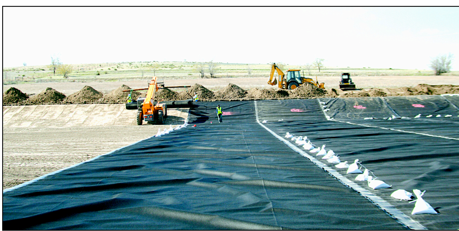
CREW MEMBERS worked to lay the black liner inside the first lagoon (above) of Oberlin's new waste water treatment plant on Thursday. One of the members used a small
