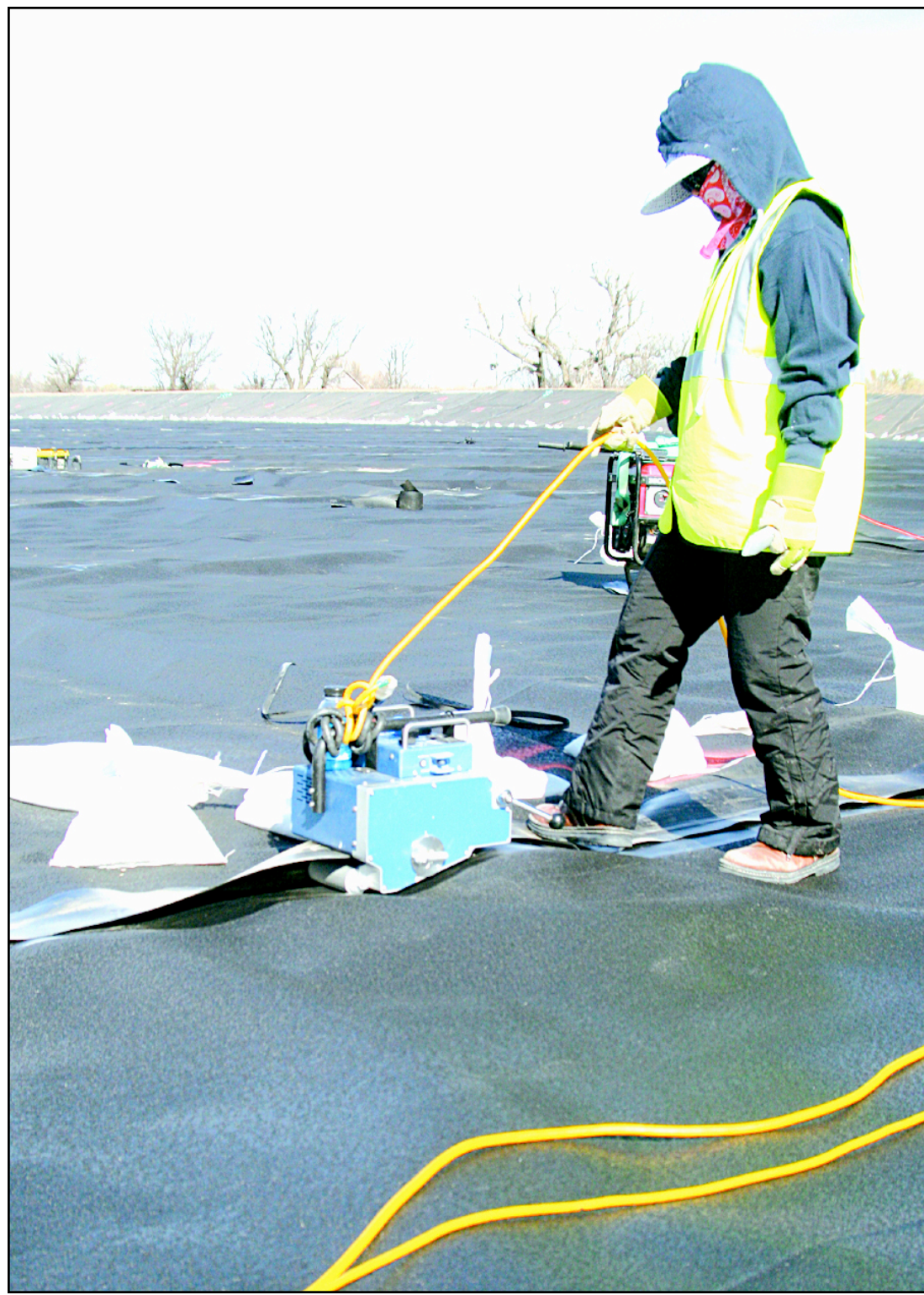
CREW MEMBERS worked to lay the black liner inside the first lagoon (above) of Oberlin's new waste water treatment plant on Thursday. One of the members used a small
