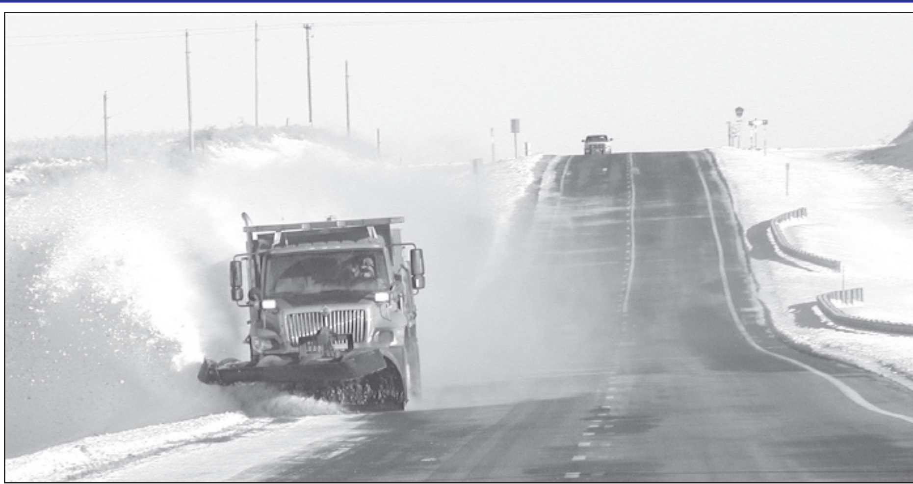
A STATE SNOWPLOW driver worked east of Oberlin on U.S. 36, scraping the snow along the edge of the pavement and starting to clear the shoulders. After a couple of days of long shifts, the crew declared victory Sunday and went home, with the driving lanes mostly dry and conditions posted as "normal" through the county. The state crew also had to clear U.S. 83 and K-38.
