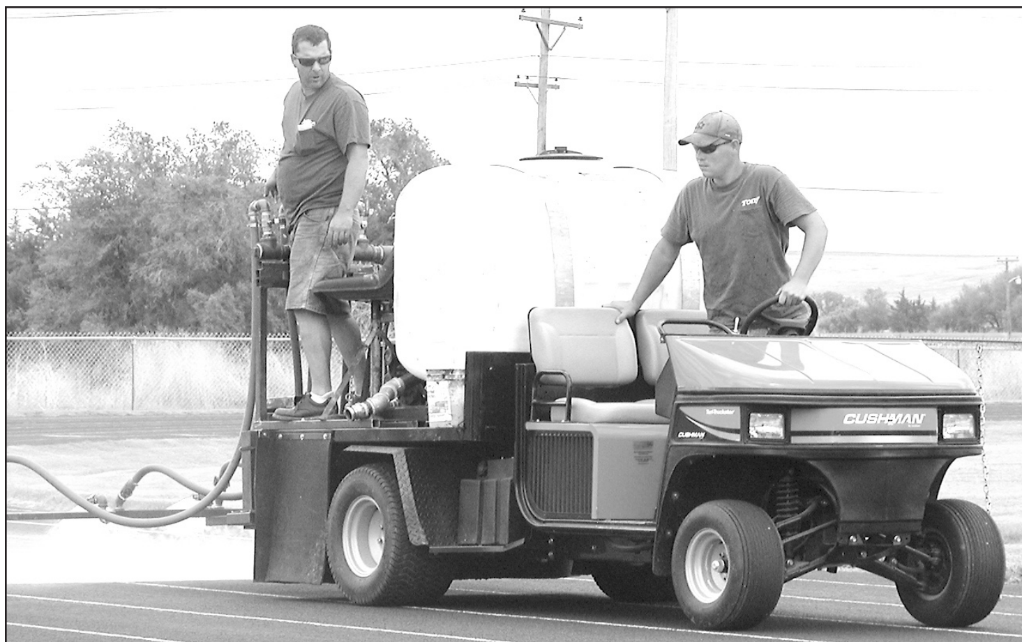
MEN WITH THE FIRM , Track Restoration out of Wichita, worked resurfacing the track at Decatur Community High School last week. Superintendent Pat Cullen said he thought the project would be done today. — Herald staff photo by Kimberly Davis
