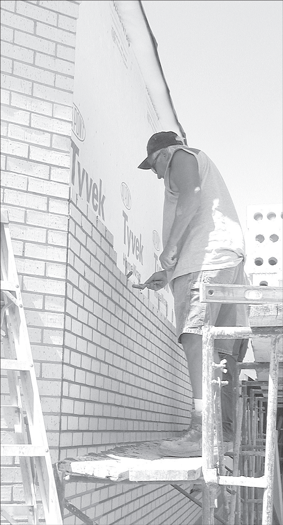
IN 2007 construction crews including Martin Pfister worked on the new speciality clinic addition at the Decatur County Hospital.
