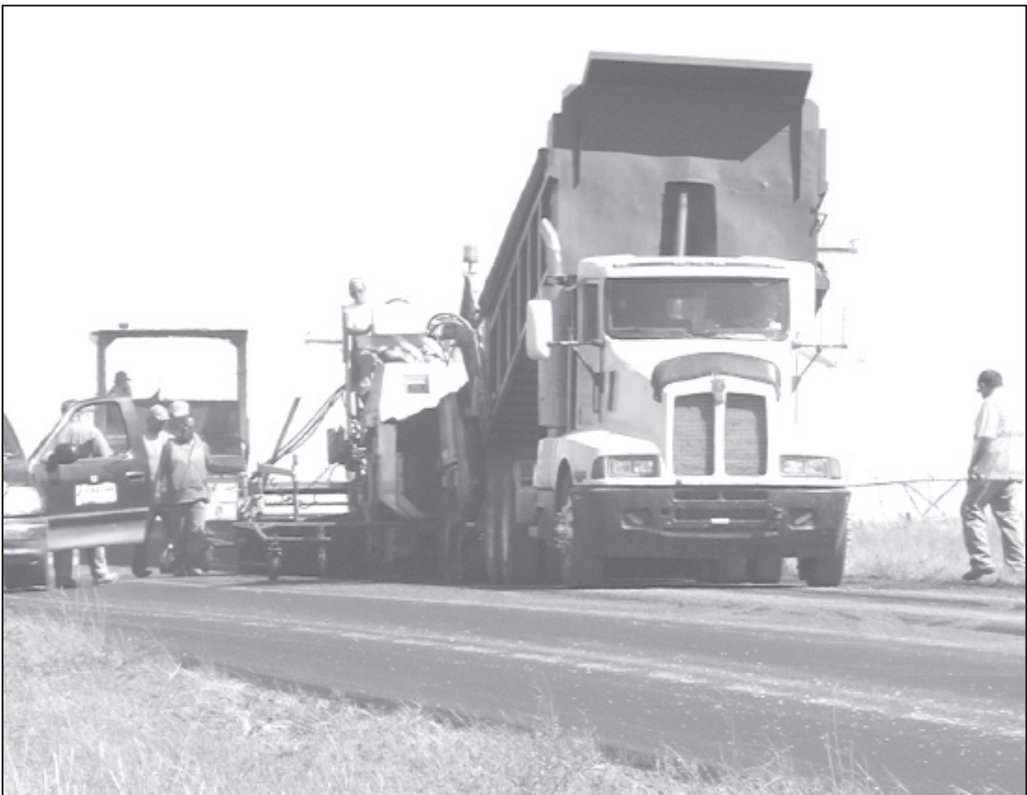
A BIG DUMP TRUCK fed asphalt to a paving machine Friday as a crew with Venture Corp. (above) worked on U.S. 83 south of town. The firm is repaving the road from
