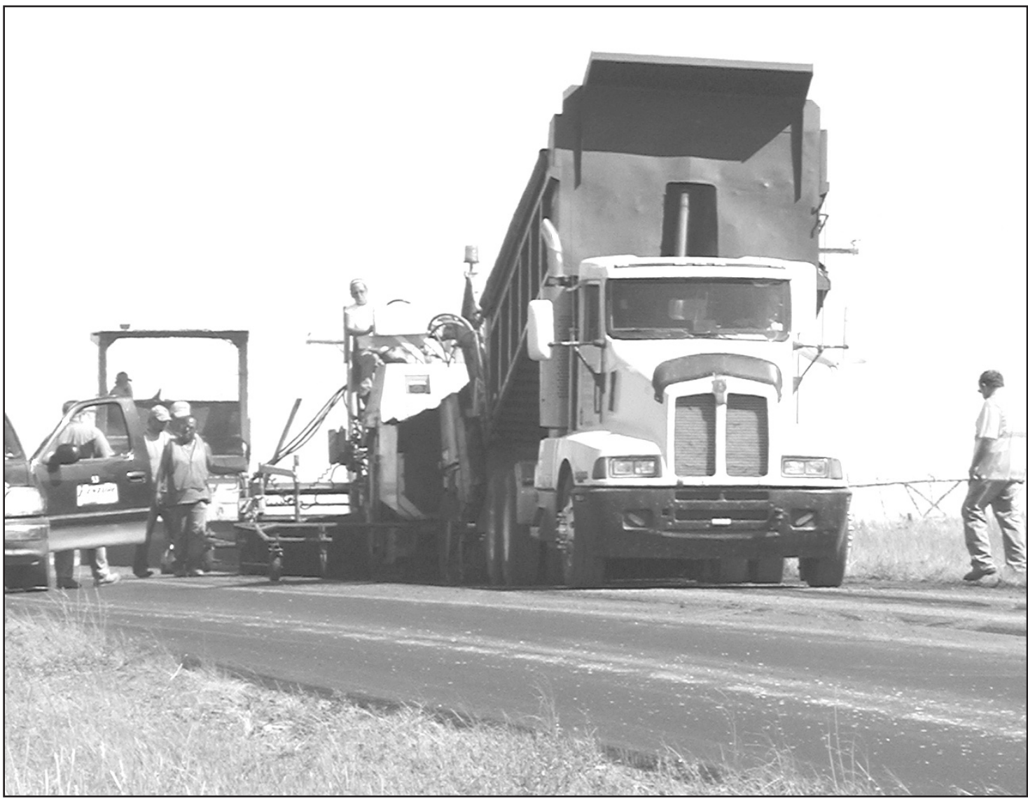
A BIG DUMPTRUCK fed asphalt to a paving machine Friday as a crew with Venture Corp. (above) worked on U.S. 83 south of town. The firm is repaving the road from eight miles south of town to the K-383 junction. Over a dozen vehicles (below) followed a pilot car through the work zone.
