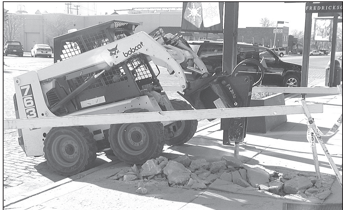
ON THE WEST SIDE of Penn Avenue, David Sporn (above) broke up concrete on the sidewalk so the city crew could replace a water line. Dan Dempewolf (left) carried a ladder to the hole on the east side of the street so the water operators could climb out.
