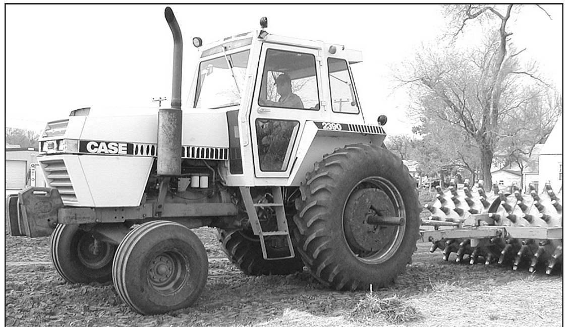
WITH A TRACTOR, another member of the crew pulled a sheep's-foot roller that packed the dirt last week.
