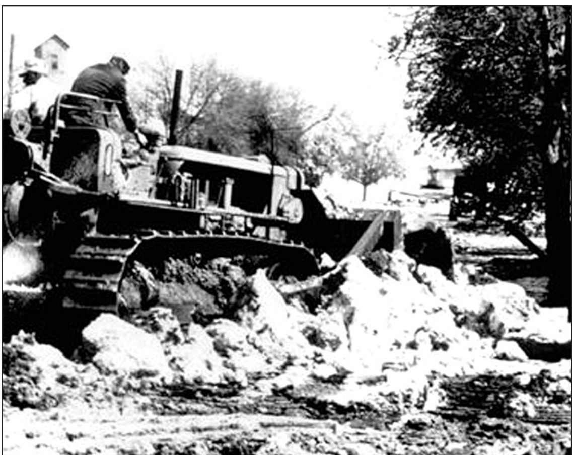
ICE WAS BULLDOZED into piles against the background of the sagging awning of the Farmers Union building in Selden. Men worked to clear hail from streets and debris from collapsed sections of buildings.
