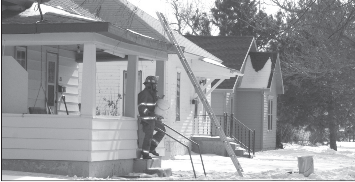
ON THE FRONT porch of a house at 211 N. East on Thursday, a fireman (above) carried a five-gallon bucket full of smoldering insulation outside. Chief Bill Cathcart
