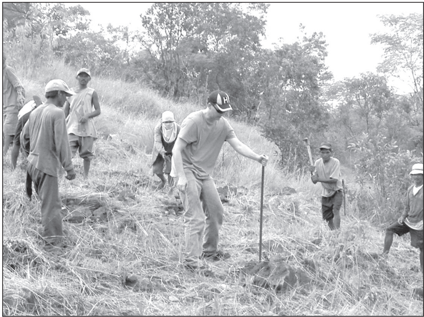
WORKERS WERE BUSY preparing the soil and building terraces for new trees to be planted near Manilla. Ward Wurm (center with shovel) spent much time helping
