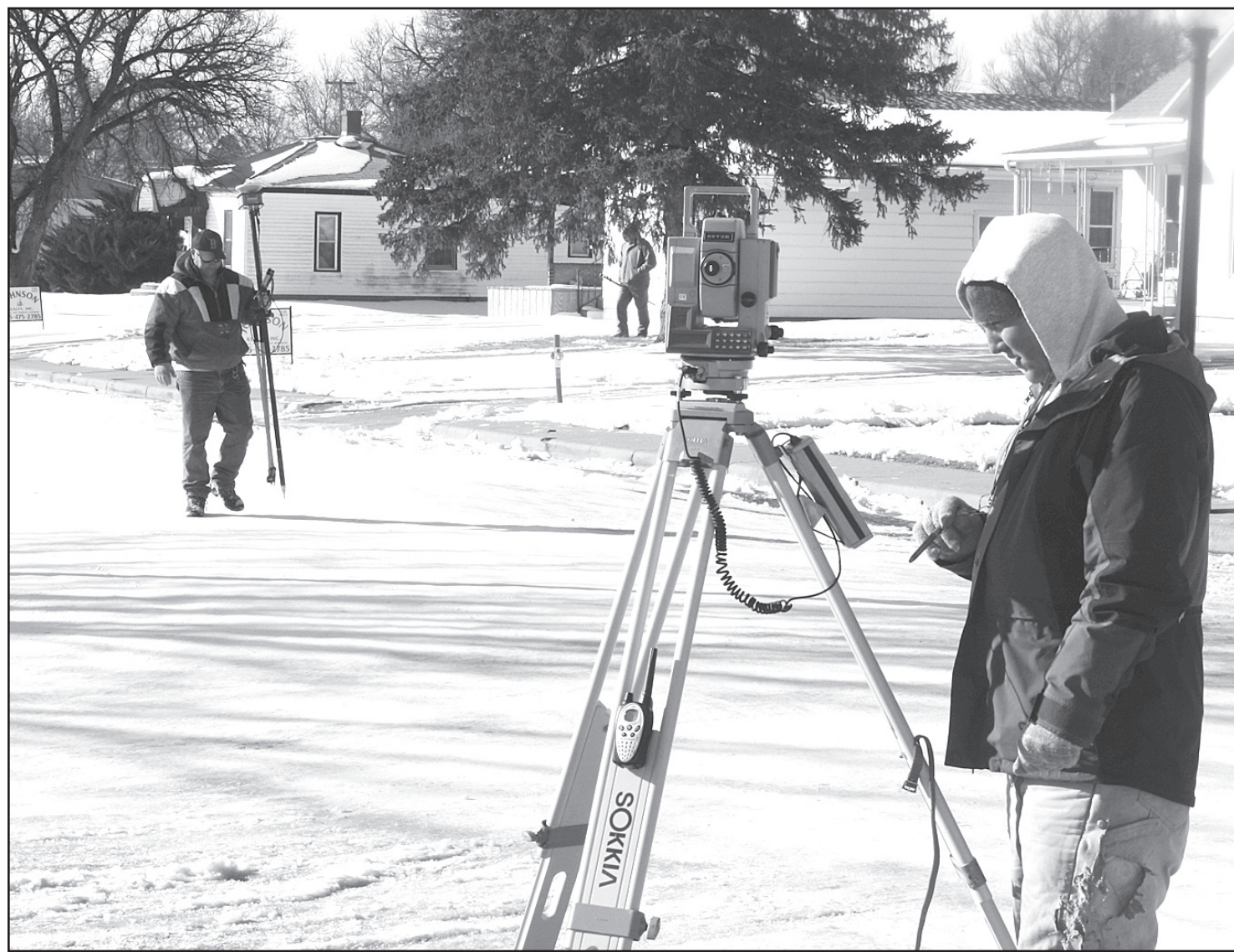
ACREW DID SURVEY WORK last week around Oberlin in preparation for building a city water treatment plant and
