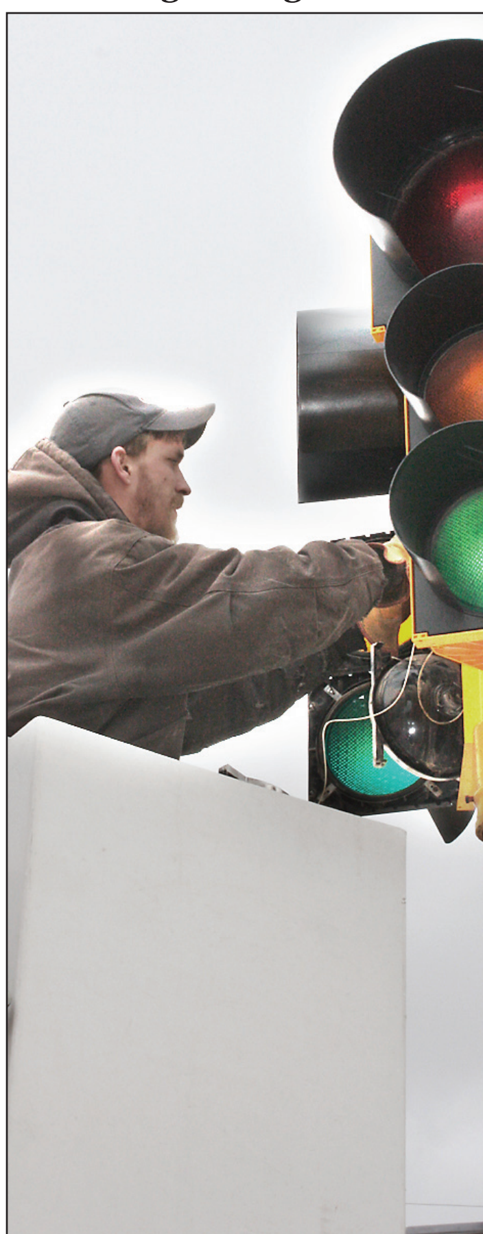
IN THE CITY BUCKET TRUCK, Dan Dempewolf replaced a bulb in a stop light at the intersection of Penn Avenue and Hall Street last week.
