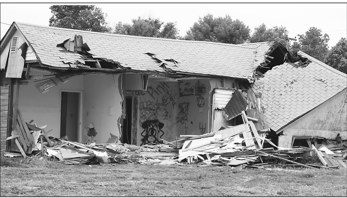
NEW OWNERS Jeff and Elizabeth Sprenkle have started tearing down the blue house at 302 W. Hall. The home, formerly owned by Nolan and Bobbi Jo Johnson, had been in the condemnation process by the city. The Sprenkles sent
