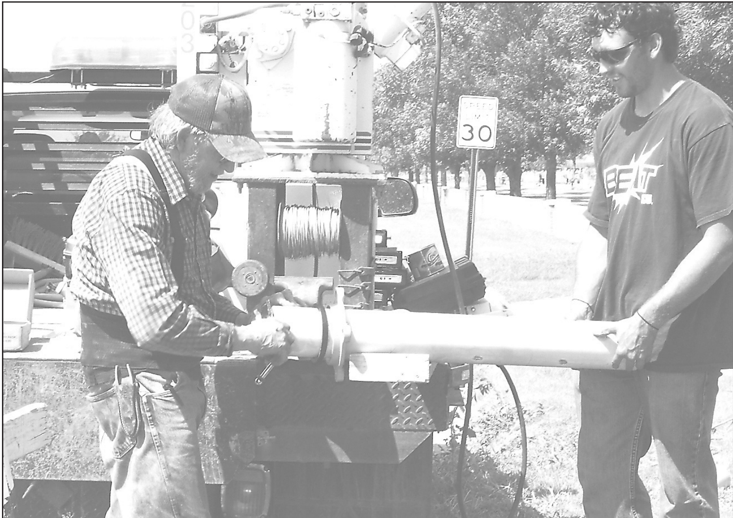
ON THE SOUTH SIDE of the city cemetery Thursday afternoon, Willard Perrin and Derek Chambers of the city water crew replaced a valve and pipe that had gone bad some time ago. — Herald staff photo by Kimberly Davis
