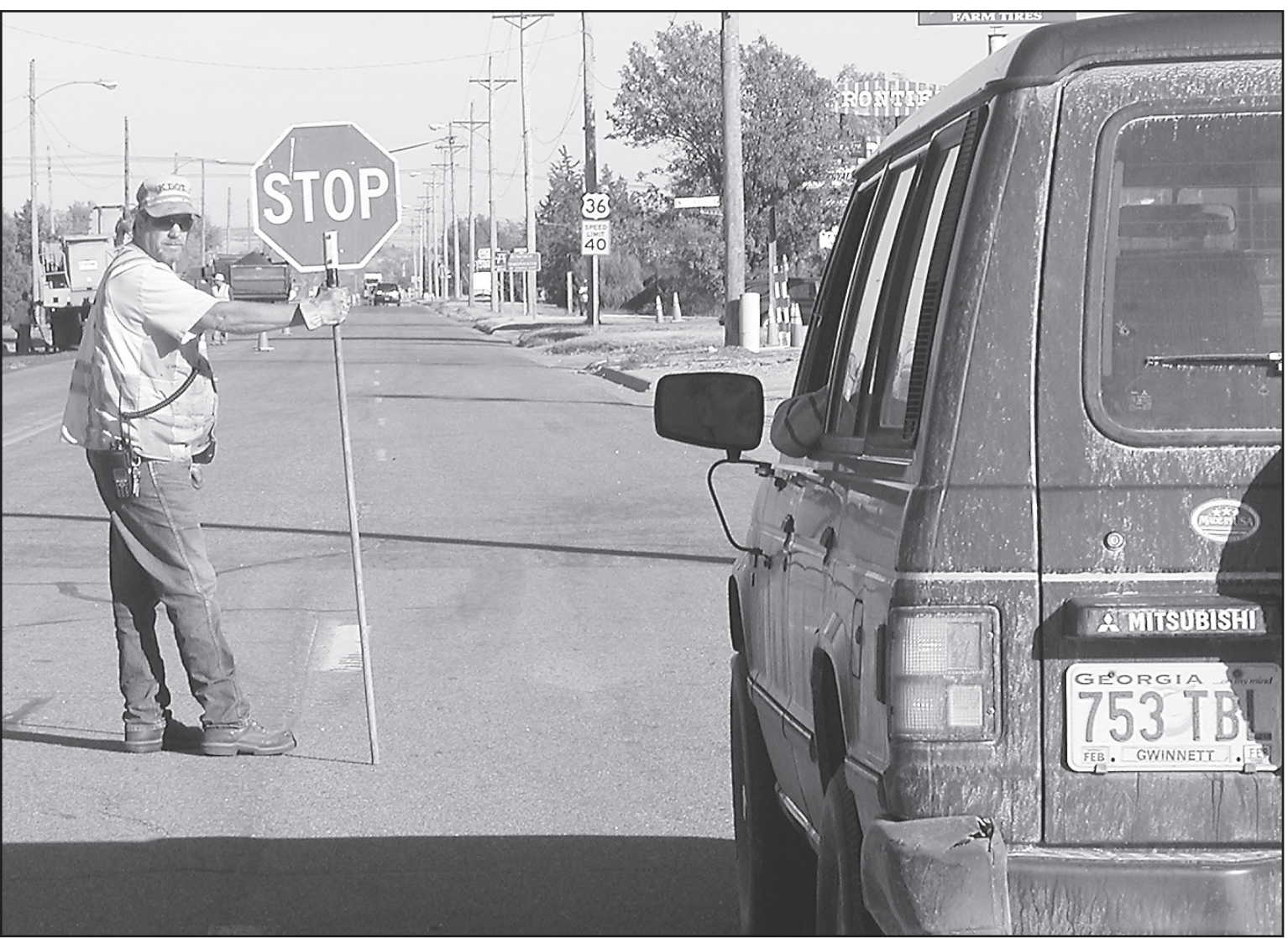
HOLDING EASTBOUND TRAFFIC , Tom Skubal of Oberlin (above) was one of the state highway maintenance workers guiding drivers around a resurfacing project on U.S. 36 in Oberlin on Monday. The crew used radios to coordinate
