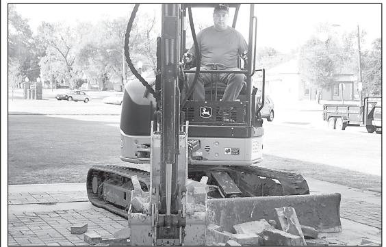
WORK ON THE ENTRANCE to the Decatur Community High School started last week. John Nelson with Nelson Concrete will replace the concrete entrance, which has deteriorated over the years. After the new porch is on, the handrails will be put back.
