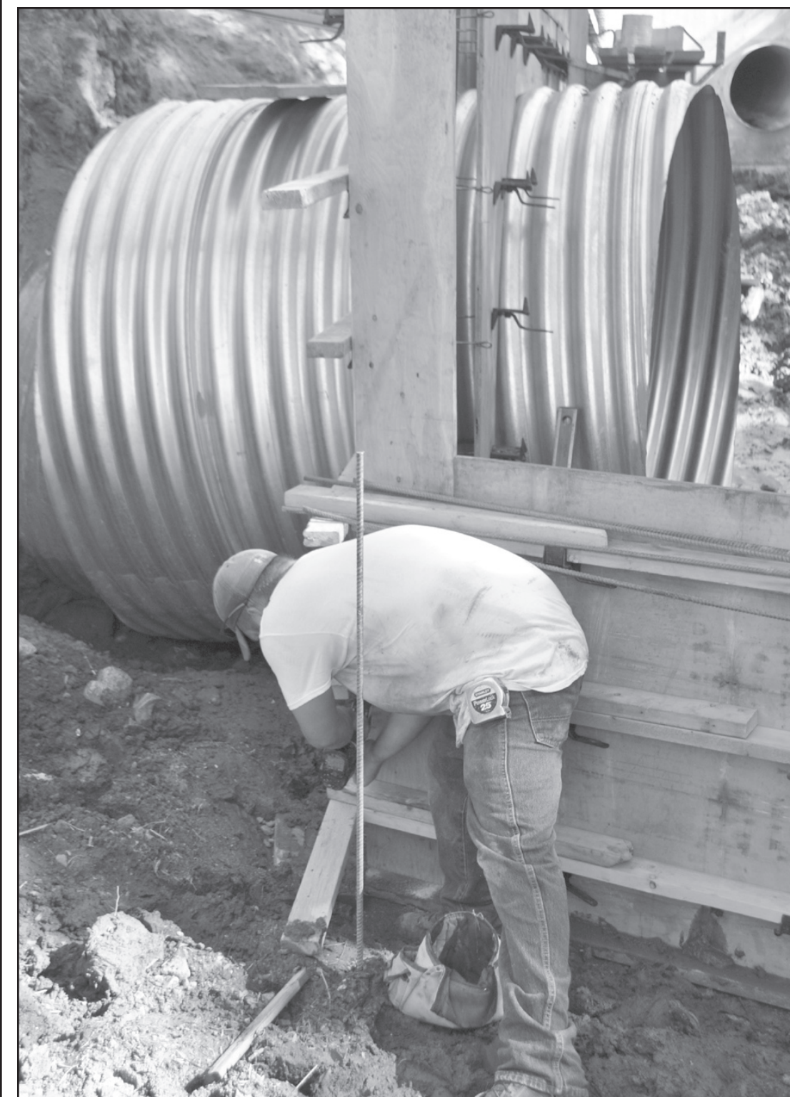
THE BRIDGE at the south end of Penn Avenue won't be done for another couple of weeks, but don't blame Nelson Concrete and Construction. The forms that Dan Fortin was working on Friday must hold concrete for a week before it's set enough to fill in behind the new wall. — Herald staff photo by Stephanie DeCamp
