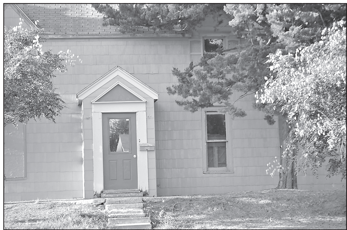
THIS PROPERTY at 203 E. Hall St. was cited by Code Enforcement Officer Jan Ackerman as blighted, but has since been refurbished through the Connections program. The program connects owners of blighted property with buyers who want to refurbish it.
