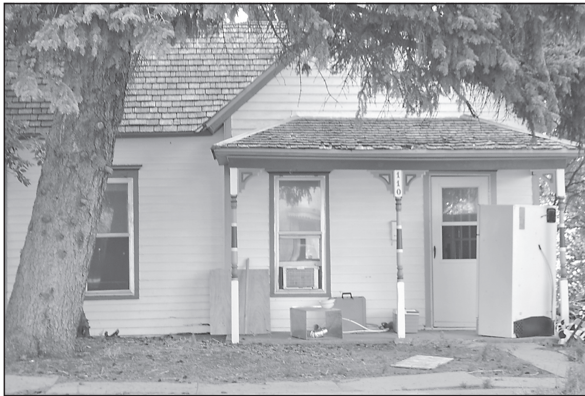
THE NEW PAINT and trim on this house at 110 S. York Ave. cleaned it up nicely after it was put into new hands, thanks to the Connections program that Code Enforcement Officer Jan Ackerman helped create.
