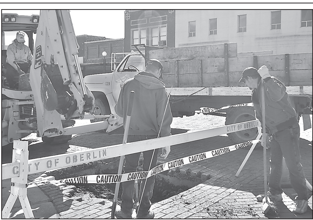
JOKING THAT THEY were digging for fishing worms, city worker David Sporn (right) looked into a hole as he and Jacob Fortin (middle) helped water department director Willard Perrin dig out an old pipe at Penn Avenue and Commercial Street on Monday. The pipe isn't in use anymore, Mr. Sporn said, and the men were just trying to eliminate a future problem. — Herald staff photo by Stephanie DeCamp
